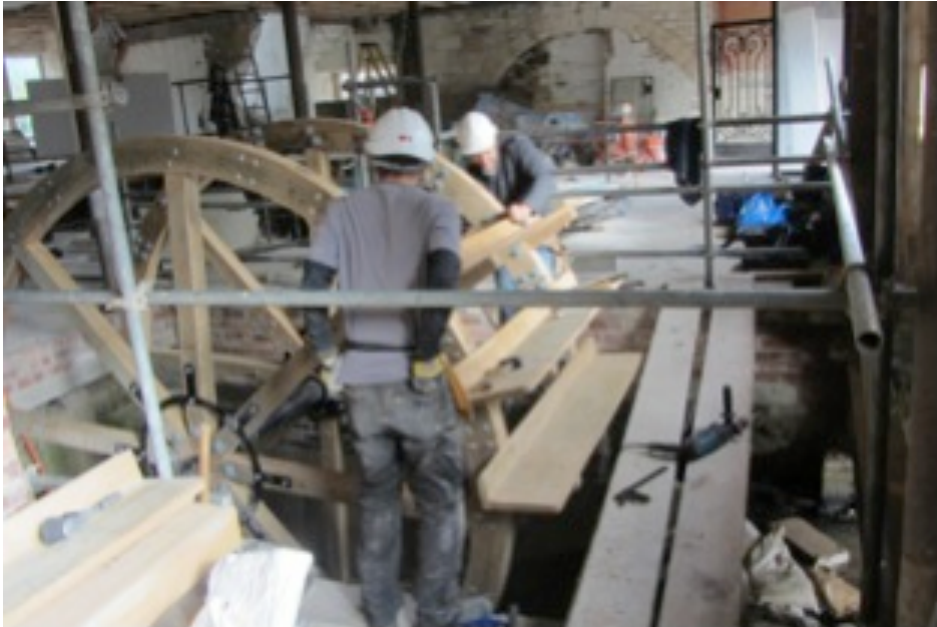
Nearing completion, with the first paddles being fitted
