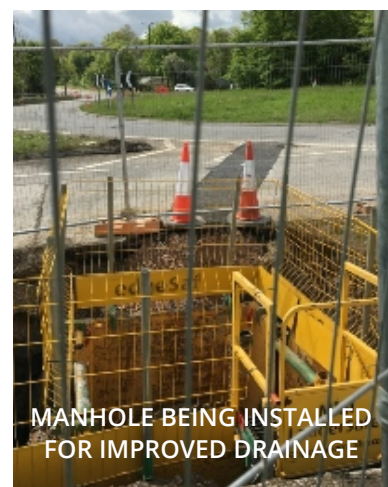
CHIPMANS PLATT ROUNDABOUT DEEP DRAINAGE WORKS
