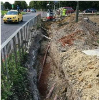
Excavation work at Old Ends Lane to uncover existing services
