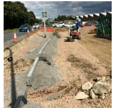
Installation of new kerb line at Old Ends Lane
